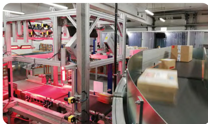
The installation of an automatic sorting system is an essential factor in speeding up the handling operations in Baunatal.
