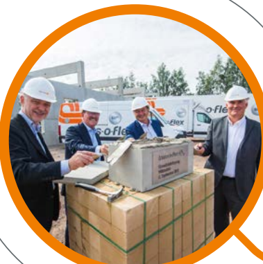
At the laying of the foundation stone for the new logistics centre, which will further increase capacity and efficiency at trans-o-flex and will be built in a very environmentally friendly way (from left): Peter Morgenroth, designated branch manager of the Wildenfels facility, Wolfgang P. Albeck, trans-o-flex CEO, Christoph Schoeller, shareholder of trans-o-flex, and Tino Kögler, mayor of the town of Wildenfels.
