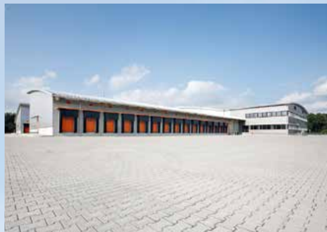
The building floorplan is not a traditional rectangle, it has the form of the letter "Y". In this way, more gates can be installed in the same space.
